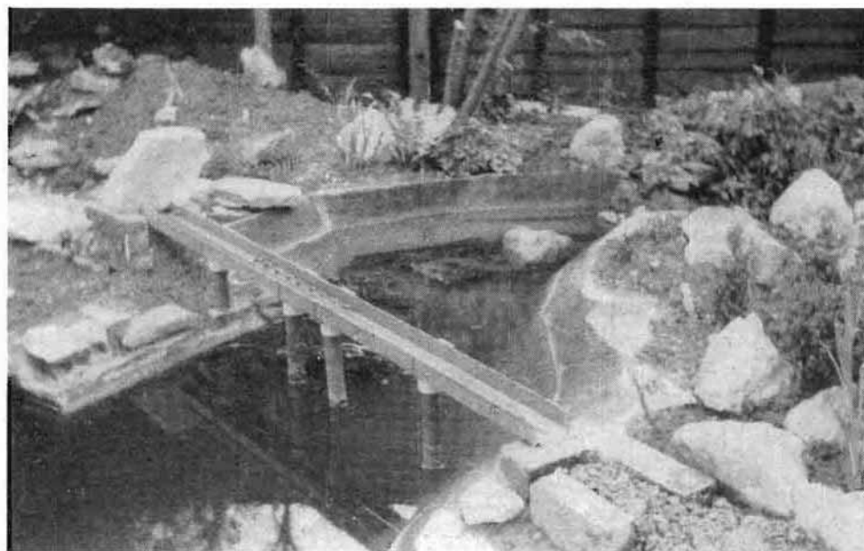
CONSTRUCTION OF BRIDGE OVER POND showing how welded angle-iron rests firmly on brick supports. Full details described in the text. Eddie Bray's pond bridge is single track.
