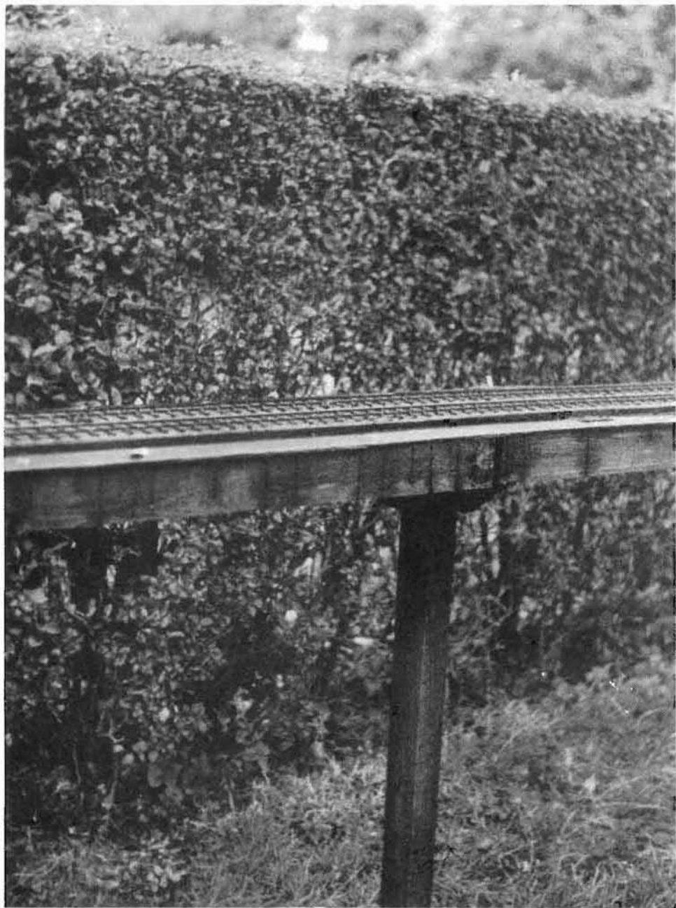
TIMBER BASEBOARD SUPPORTS by Deryck Featherstone. Oak Post into ground. Finescale Gauge '0' track on asbestos baseboard. Although narrow, room is left for signals, fencing, etc. In use 20 years when photographed! Photo: D. Featherstone.
