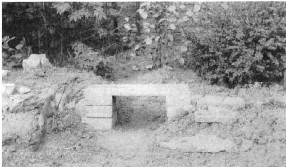
BUILDING AN UNDERBRIDGE on E. Bray's LNWR garden line. The resemblance to what goes on in reality should be noted. Piers already stone-faced to hide bricks.
